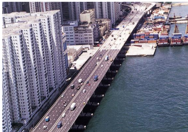
Figure 2: First PMFC trial on high speed road in Hong Kong
